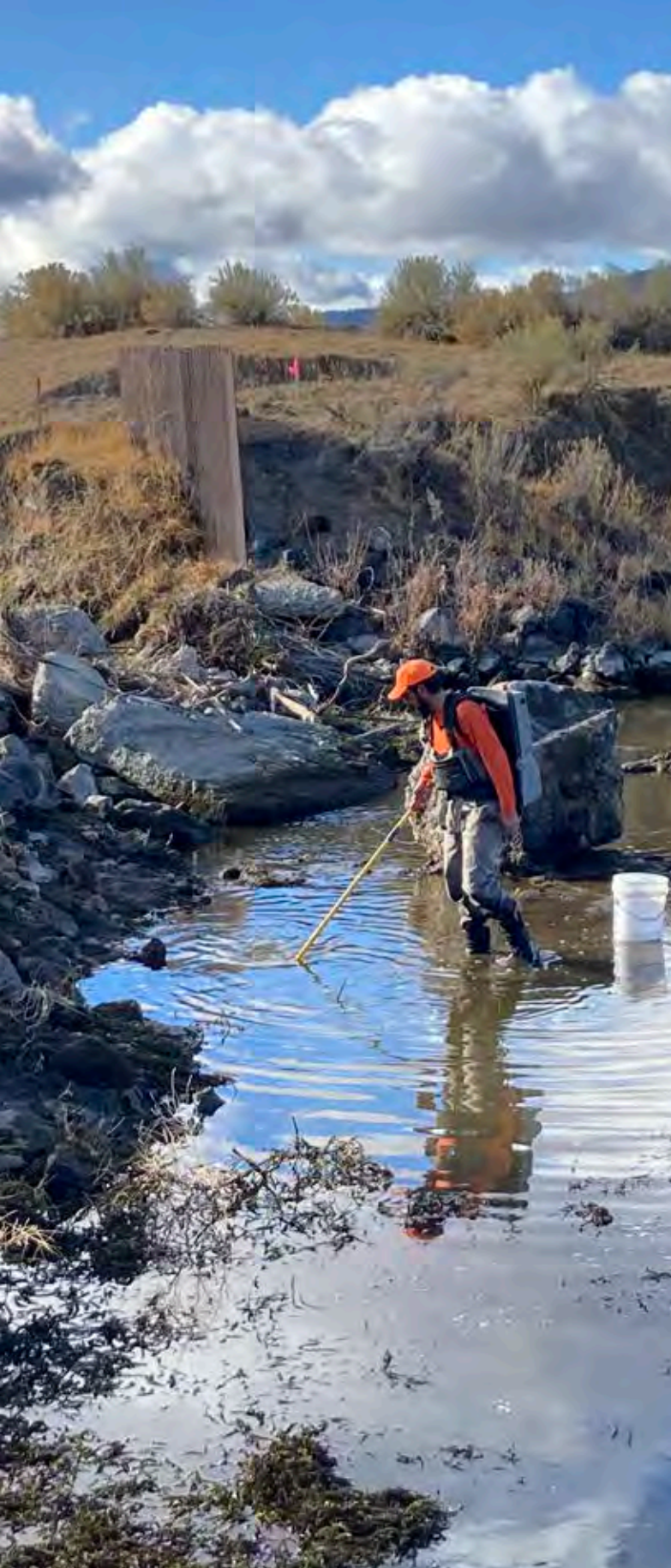
Warner Basin Aquatic Habitat Partnership – ODFW Fish Biologist Justin Miles doing fish salvage before Relict Diversion Construction. PHOTO / BRANDI NEIDER
