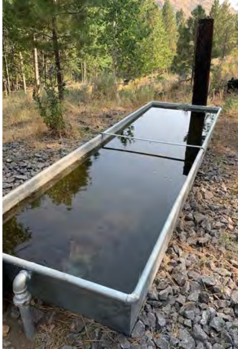
Oregon Model to Protect Sage-Grouse – Spring development trough with wildlife ramp. PHOTO / LAKE COUNTY SWCD
