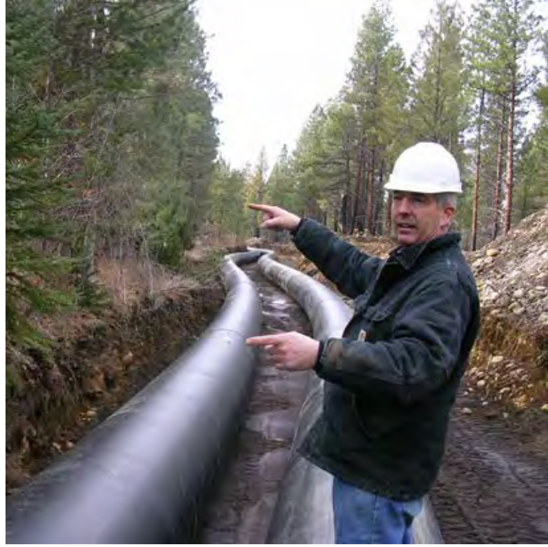
Deschutes Basin Partnership - Three Sisters Irrigation District Manager Marc Thalacker oversees canal piping, enabling flow restoration in the Creek. PHOTO / DESCHUTES RIVER CONSERVANCY
